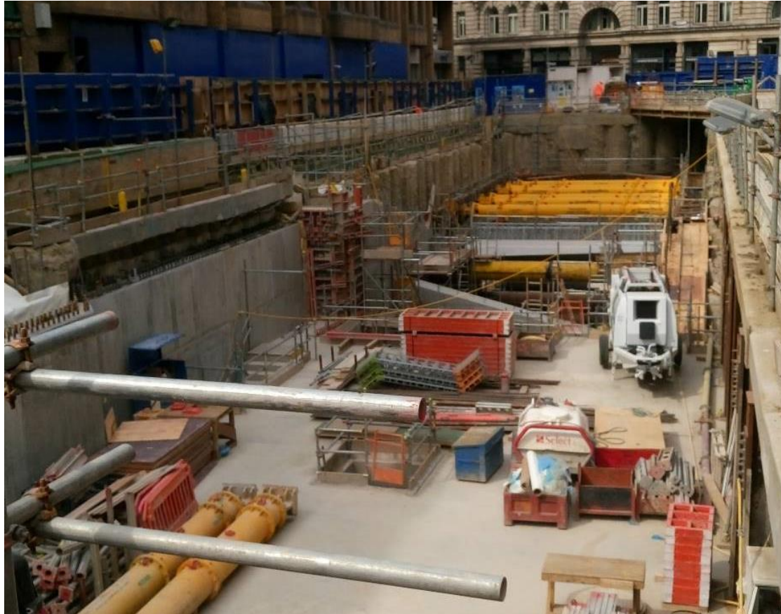
Liverpool Street Station site, London, 2016
